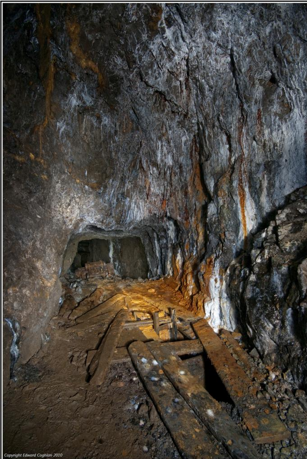
Looking at the top of the Man way and the ore shoot
