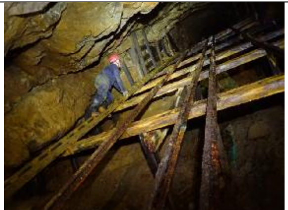
The railway incline in Tywarnehayle Mine
