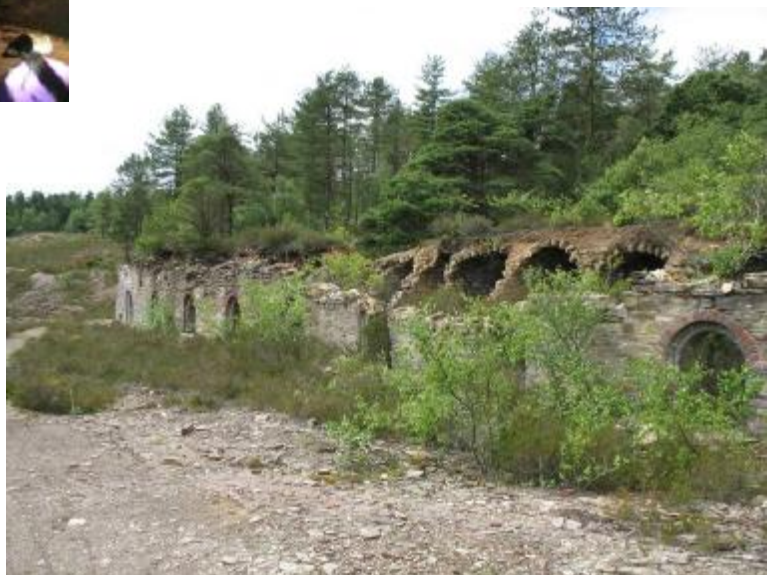
Figure 4: (below) arsenic flues at Devon Great Consols
